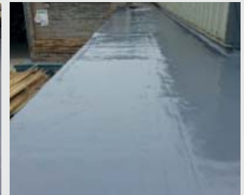
Existing Bituminous felt roofs
